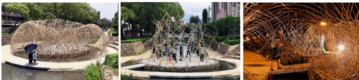
Figure 2: A digitally fabricated bamboo structure featuring spiraling forms and smooth curves that blend seamlessly with the surrounding landscape (Myers, 2019).
