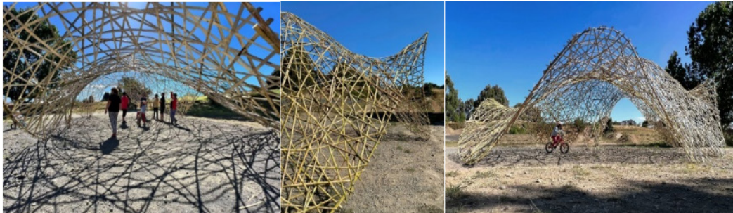
Figure 3: A mid-tech bamboo structure exploring Colihue's structural and aesthetic potential, functioning simultaneously as both envelope and framework through its flexible, versatile form (PA Editorial Team, 2023).
