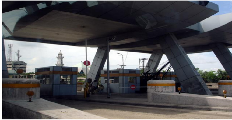
Figure 3: Proposed area (Meghna Bridge Toll Booth)
