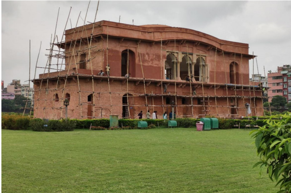
Figure 10: Ongoing Conservation Project (Source: Author)
