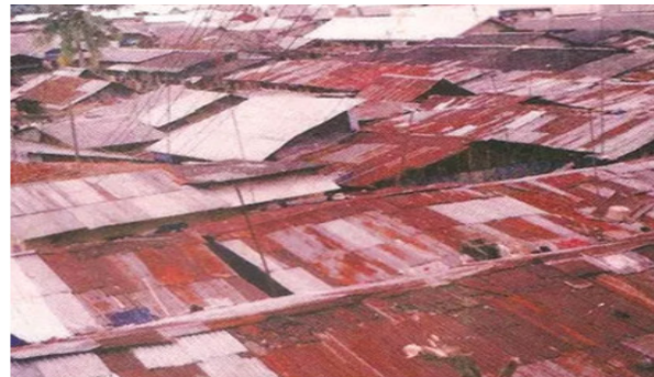
Figure 6: Corroded Building Roofs with Acid Rain in Oporoma
