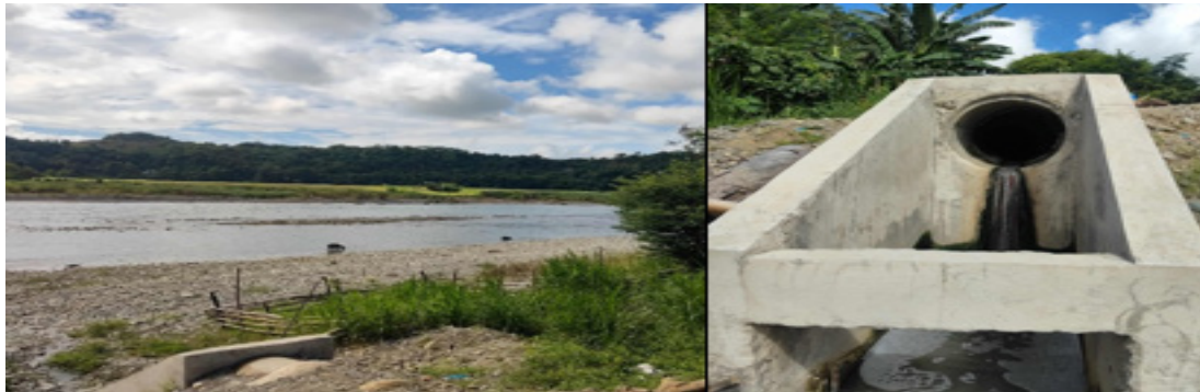
Figure 12: Drainage directly discharging wastewater beside Station 6
