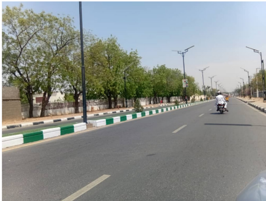
Figure 5: A section of Ahmadu Bello Road showing effective road infrastructure with smooth surfacing, clear markings and street lighting. Source: Fieldwork (2025).
