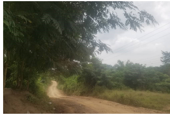
Figure 1: The 3rd class road which leads to Wuruduwurudu. Personal picture taken by consent of the headteacher.
