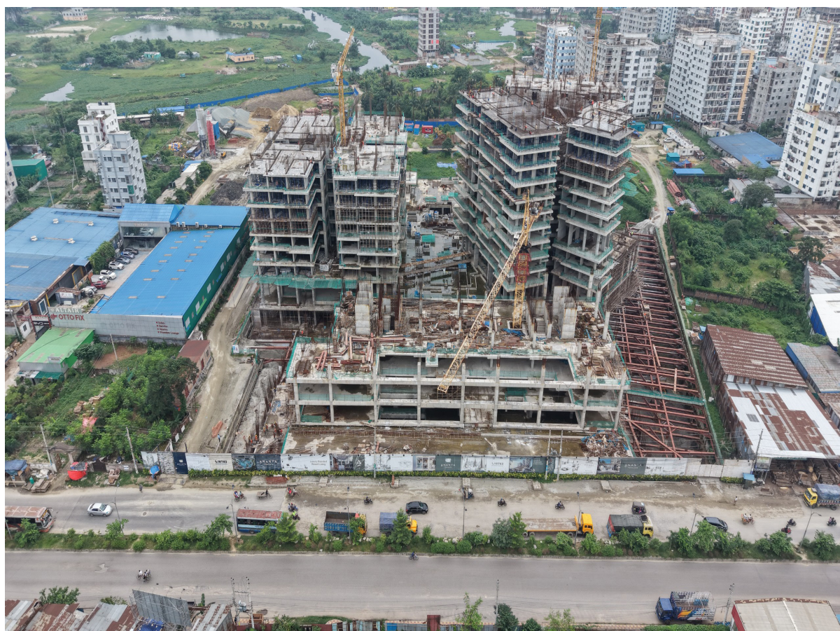
Figure 1: Top-down drone view of a multi-tower high-rise residential project under construction in Dhaka, illustrating simultaneous superstructure progress across towers, active tower-crane operation, and site logistics. Image captured June 2026.
