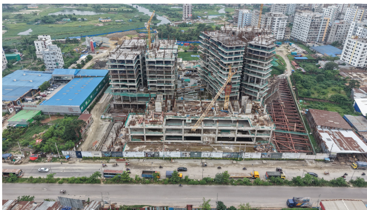
Figure 1: Top-down drone view of a multi-tower high-rise residential project under construction in Dhaka, illustrating simultaneous superstructure progress across towers, active tower-crane operation, and site logistics. Image captured June 2026.
