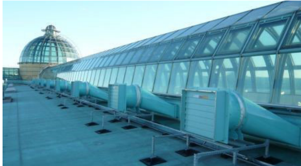
Figure 1: System for Controlling Smoke.
